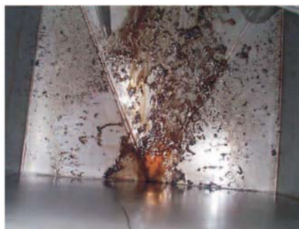
Figure 14. The bottom of a tank in a hydraulic system, equipped with a 3\mu\text{m} (beta value 200) inline filter.
